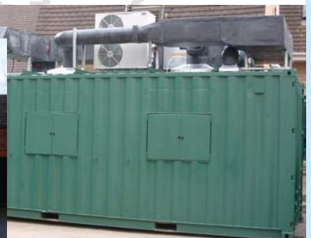
6m Reinraum-Container, Yorkshire Clinic
